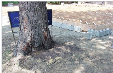
Foundation is very close to this maturing tree. Photo: Andrew Koester, International Society of Arboriculture, Bugwood.org
