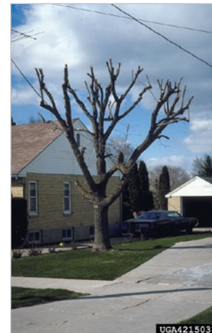
Trees and powerlines do not mix! Photo: Fred Baker, Utah State University, Bugwood.org
