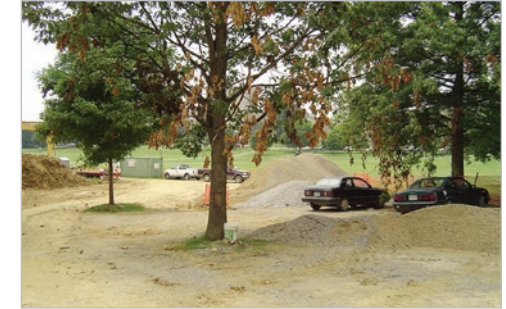
Top soil removed and subsoil compacted around the bases of the tree. Photo: Eric Wiseman, Virginia Tech
